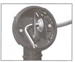
For power connection applications: Install power connection fittings (user supplied) and pull in power and ground wires.
